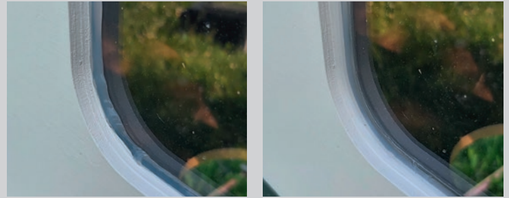
Smoothed silicone joint
